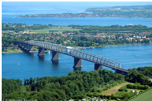
Figure 1. The old Little Belt Bridge is 1.178 metres long and 20.5 metres wide. The passage height is 33 metres. Fyn is seen in the distance. Photo: H.C. Steensen.
