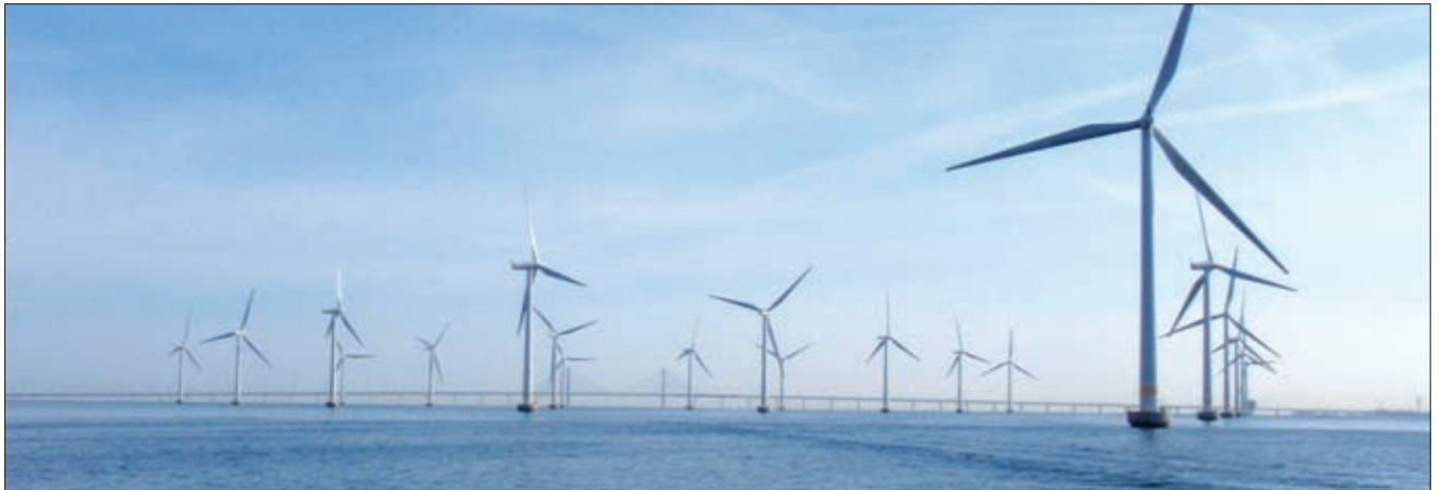
GEO has carried out site investigations for more than 35 offshore wind farms
